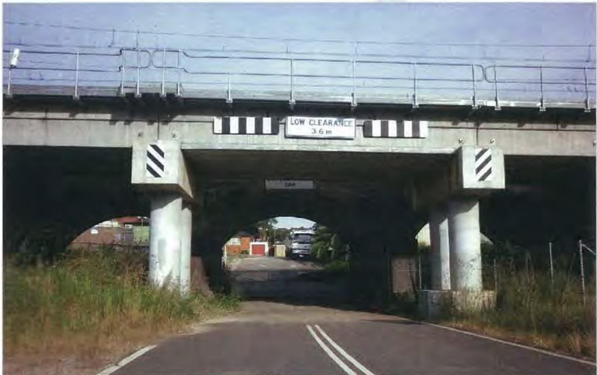
Figure 4.0: Woodbrook Road Underpass (looking from Powerhouse Road, toward east)
